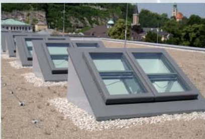
Mounted on a sloped plinth
