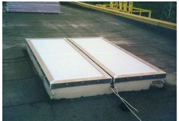
Replaced with weather-resistant polycarbonate multi-seamed hoods while retaining the control system.
